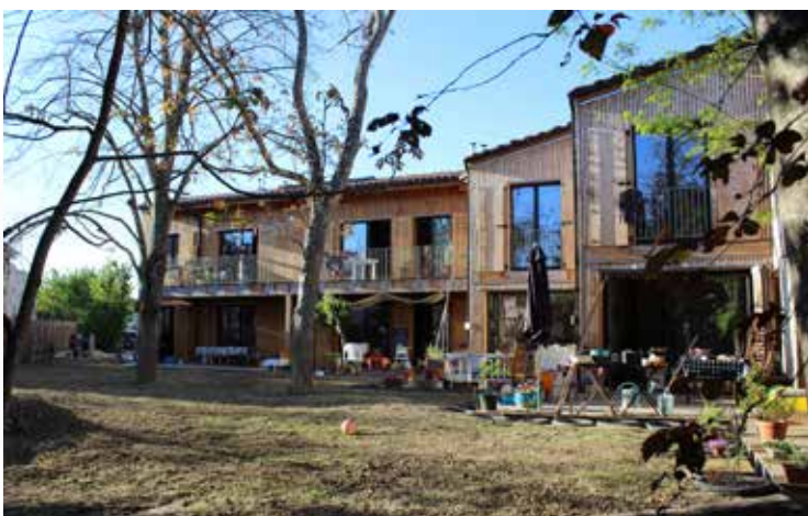
Façade sud. - Photo © MC Couthenx
